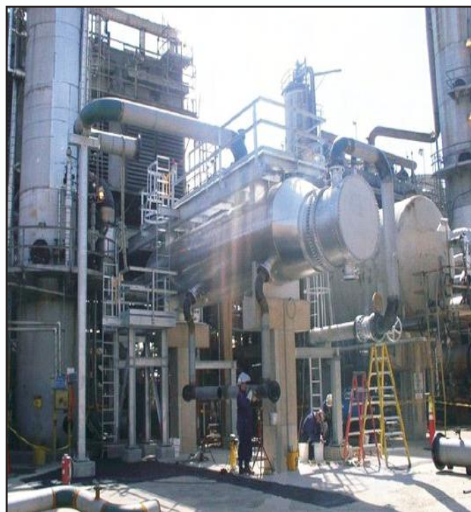
Revamping of SWS Unit at the CPCL, Chennai
