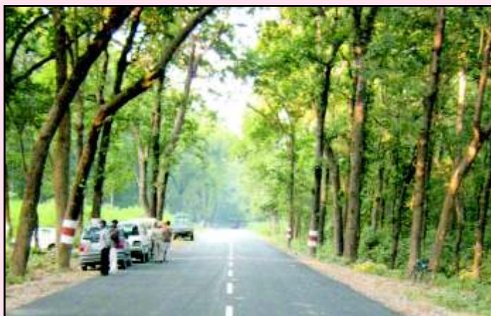
A view of the test road section on the Delhi-Yamunotri road at Km No 223-224
